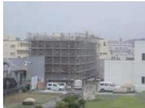
The status of construction work at the high-voltage electricity ward
