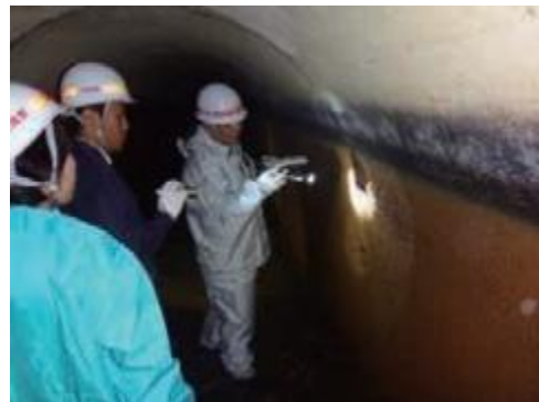
Inspection survey of the interior surface of the eastern route headrace tunnel
