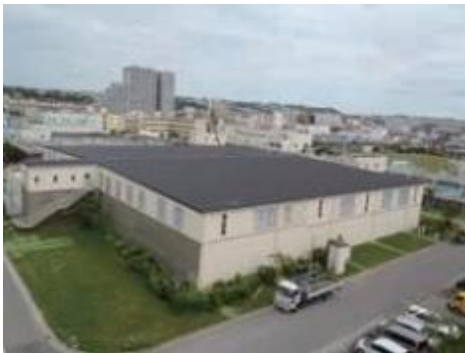
After the improvement of sedimentation basin
