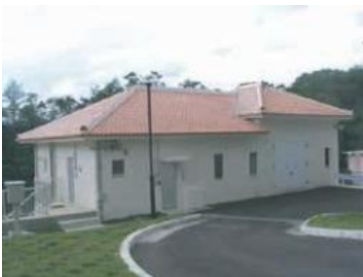
Hijagawa Water Intake Pump Station (Kadena)
