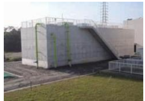
Development of an activated carbon treatment facility (newly constructed)
