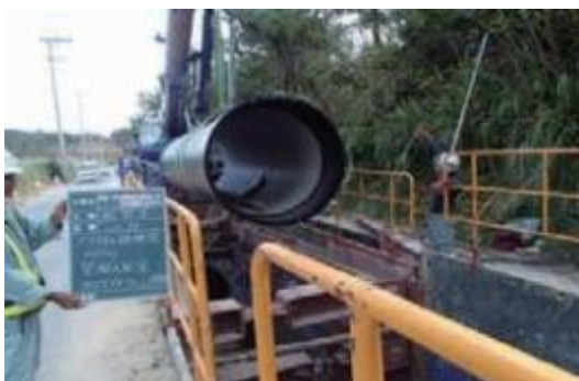
Construction of the water conduit between Fukuji and Udenaha
