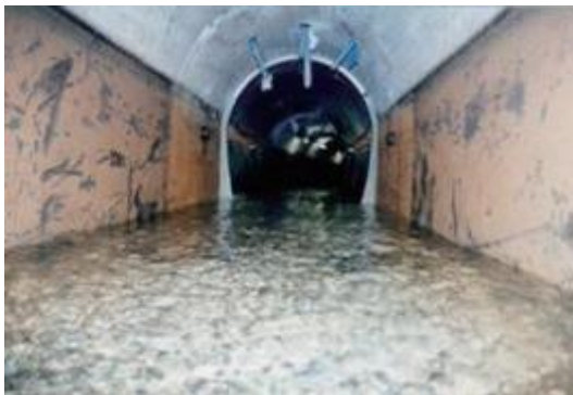
Interior surface of the eastern route headrace tunnel
