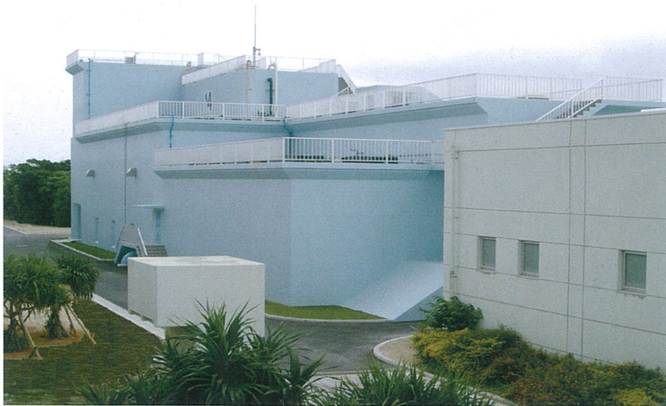
Water Softening Facility
